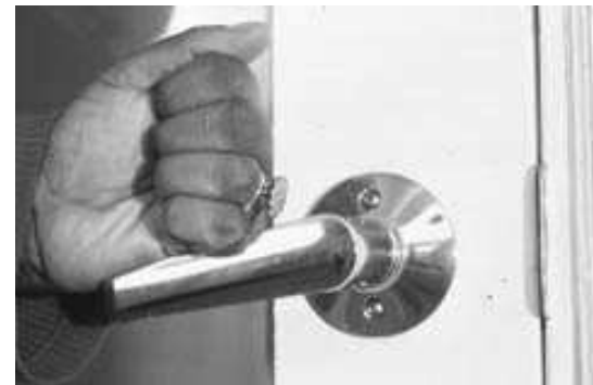
A hand with closed fingers operates a lever door handle by pushing down.
